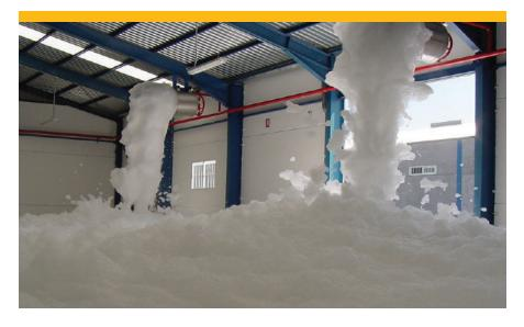
(CAFS) in class A and class B fires, where its high efficiency reduces the water consumption.
